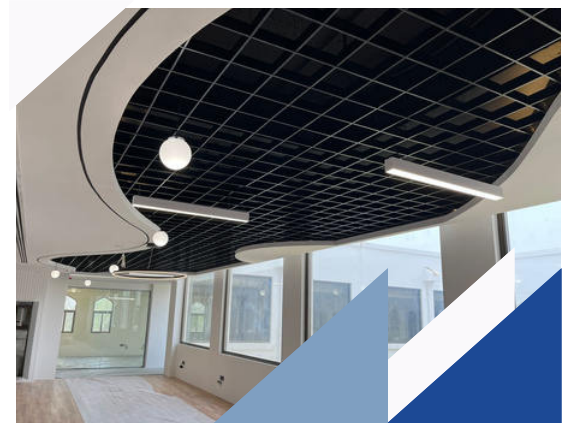
Supply and installation of interior lights at office of Ministry of Endowment & Religious Affairs - Muscat - 2025
