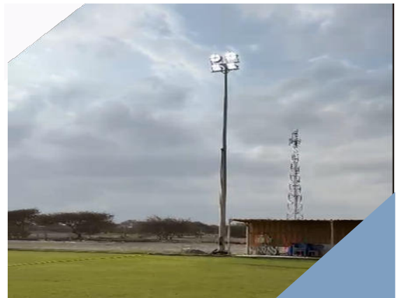
Supply and installation of Highmast light at Khabura Stadium-2025
