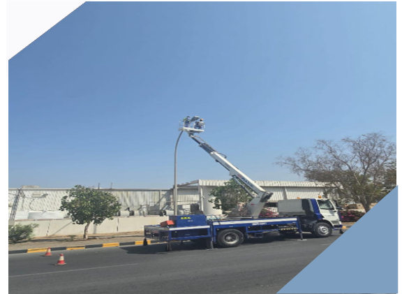
Supply & installation of Smart Street light -Madayn Industrial Estate-Muscat -2026
